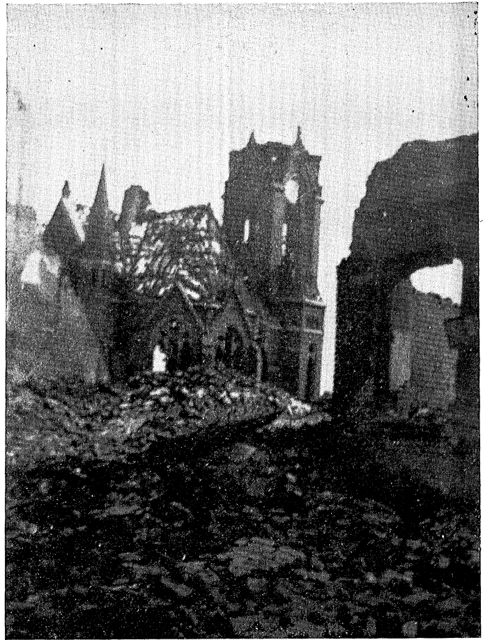
Damaged buildings in Plauen
