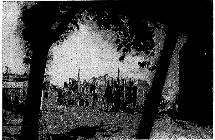
Another scene of destruction in Germany.
