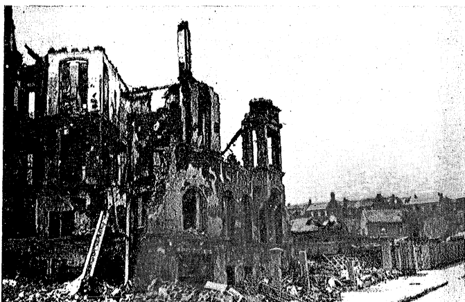
Destruction in Plauen, Germany—June, 1945.
